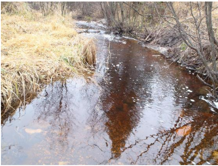
Lost River Rock Weir
